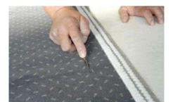
repeats match. Each individual roll edge is precisely to be cut according to the pattern repeat in the tuft channel, pattern line, or parallel to the print edge.
